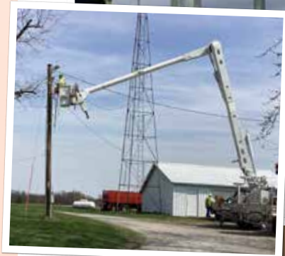
Crew working on a member's service.
