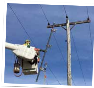
Crews working on 3-phase services.
