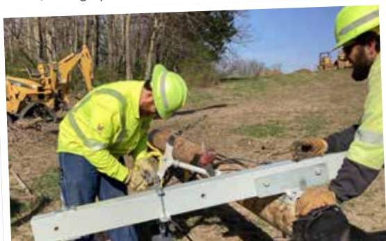
Crews framing a pole.
