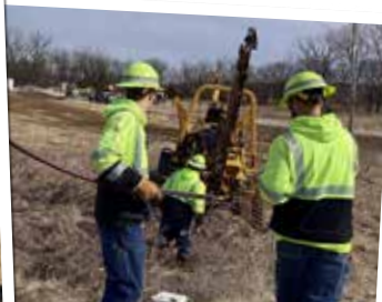
Crews trenching a primary underground service.
