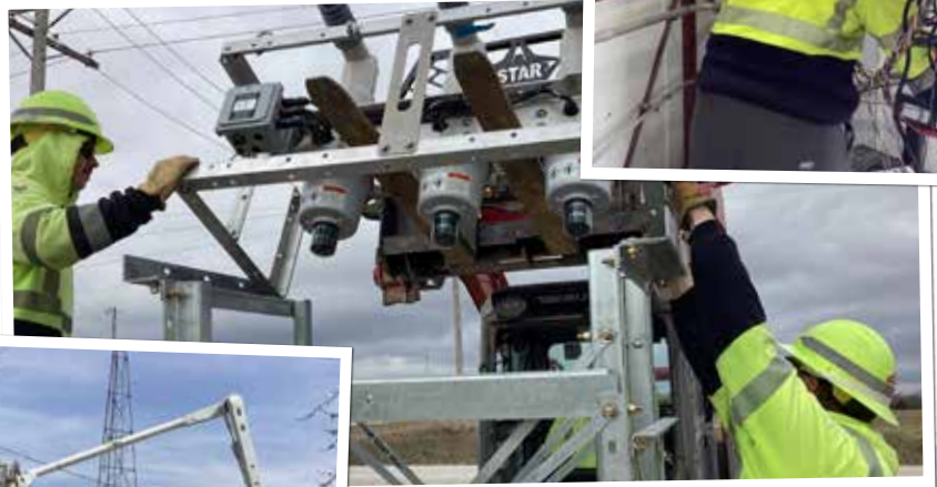
Crew installing a new substation recloser.
