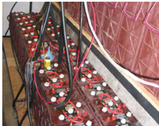
▲ A battery bank
