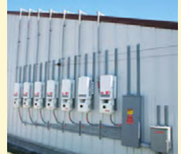
▲ A set of string inverters
