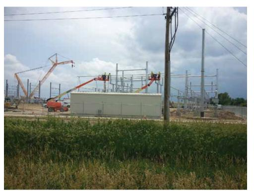
Construction continues at the lowa Fertilizer Company near Wever. Northeast Power is working with Access Energy Cooperative crews on building the substation that will provide power for the plant.
