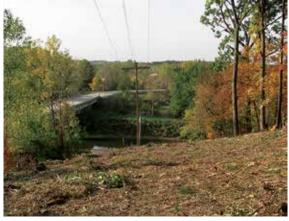
Specifications can vary, but a general guideline of maintaining a safe ROW is 15 feet of clearance on either side of the primary conductors and 20 feet of overhead clearance above the highest wire on the pole.
