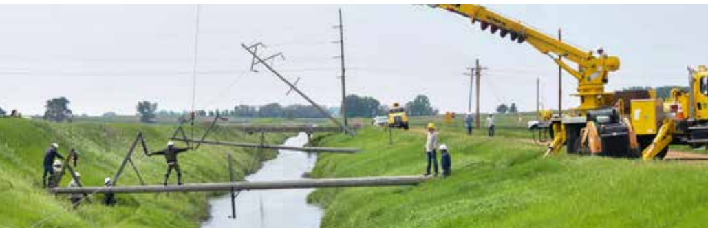
◀ Corn Belt Power Cooperative transmission crews cleared downed structures, phases and equipment on May 22 before rebuilding this stretch of line northeast of Farnhamville.
