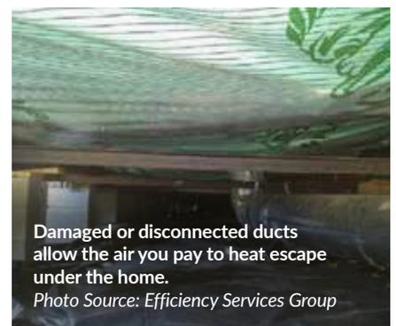
Damaged or disconnected ducts allow the air you pay to heat escape under the home.
