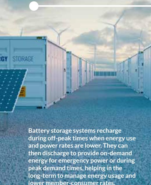
Battery storage systems recharge during off-peak times when energy use and power rates are lower. They can then discharge to provide on-demand energy for emergency power or during peak demand times, helping in the long-term to manage energy usage and lower member-consumer rates.
