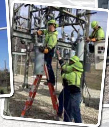
Substation recloser project to strengthen the cooperative's reliability.
