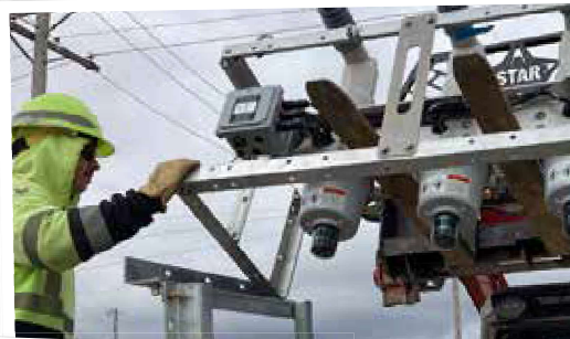
Crew installing a new substation recloser.
