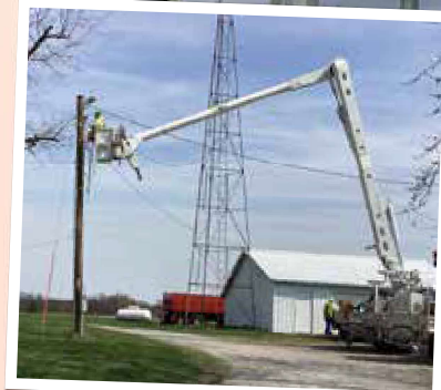
Crew working on a member's service.
