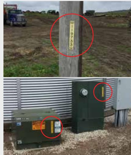
the tags are on a pole, they are usually mounted approximately 5 feet above the ground line and face a road or driveway. Ground-mounted equipment will have tags on the lid or door next to other warning stickers.
